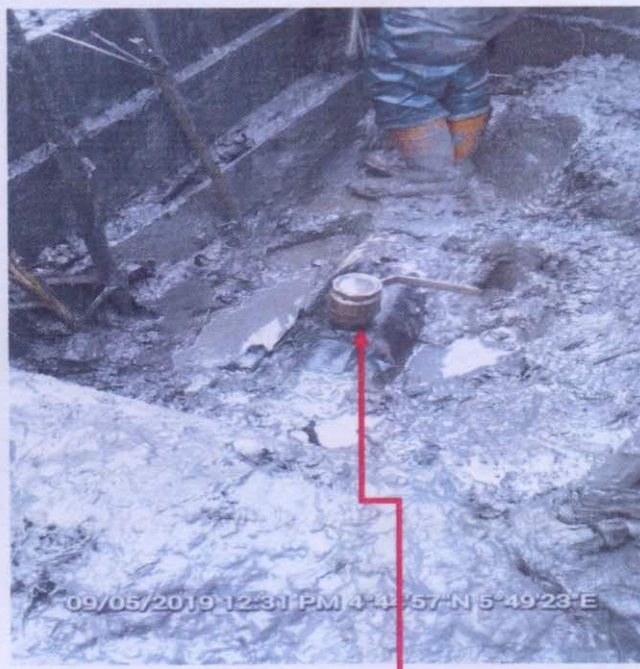
Fig B: The Incident Facility after excavation
