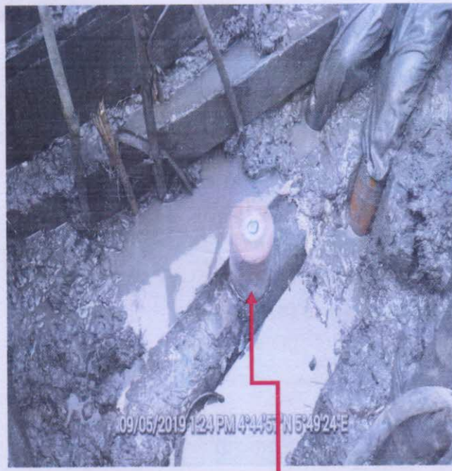
Fig C: Incident Facility during repair
